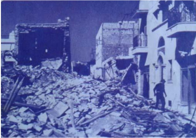
Picture 1. Earthquake Damage in Agadir, 1960 (p 16)
