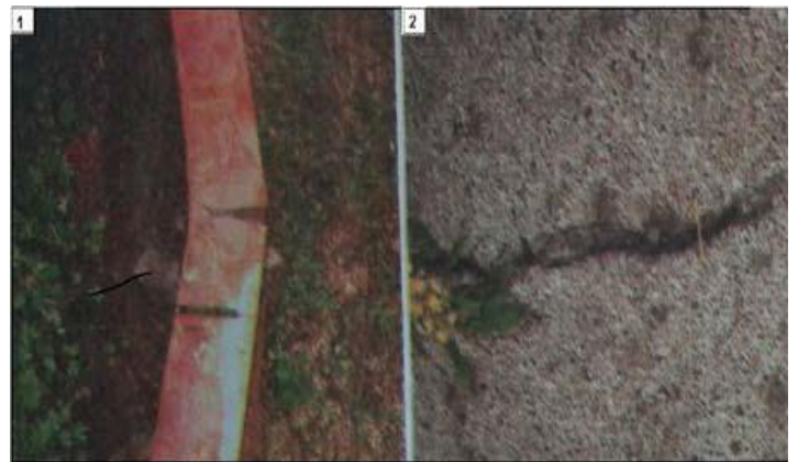
Picture 4b. Earthquake Damage in Al Hoceima Imzouren (p 21), (4b1): Deformation in the garden corridor (4b2): Appearance of cracks in a paved road (Harfani and Cherkaoui Institut scientifique Rabat).
